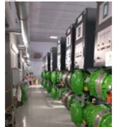
Figure 15: 420 kV GIS using g 1 installed in RTE's Gerswiller substation in 2016.
