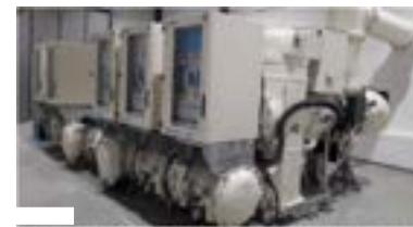
Figure 14: 120 kV GIS with g 1 installed and integrated at Rapp's E-test substation in 2016.
