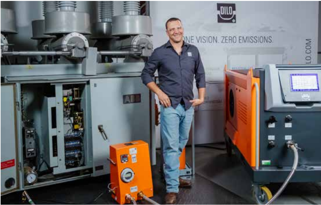
Gas handling equipment operated by trained professionals ensures zero emissions
